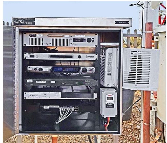
Fig. 8 LPFM system installed in weatherproof rack
