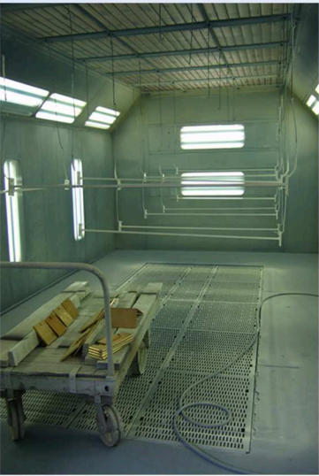
EPA/OSHA COMPLIANT PAINTING FACILITY
