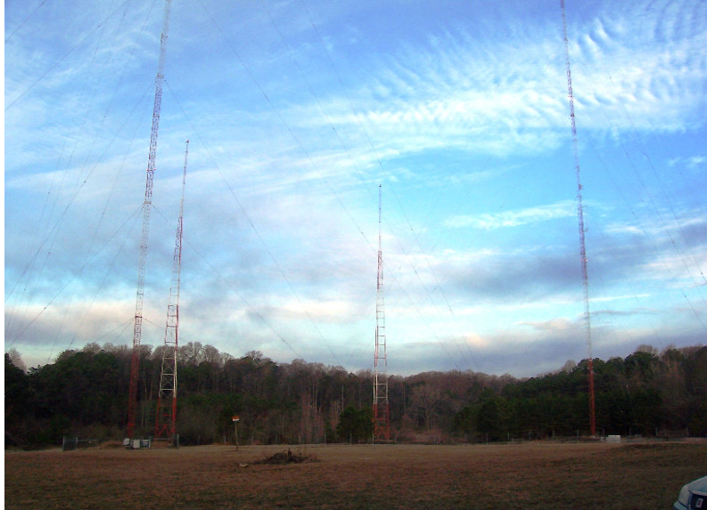
FIGURE 10. A photograph of the WAOK four-tower array consisting of two guyed and two self-supported towers.
