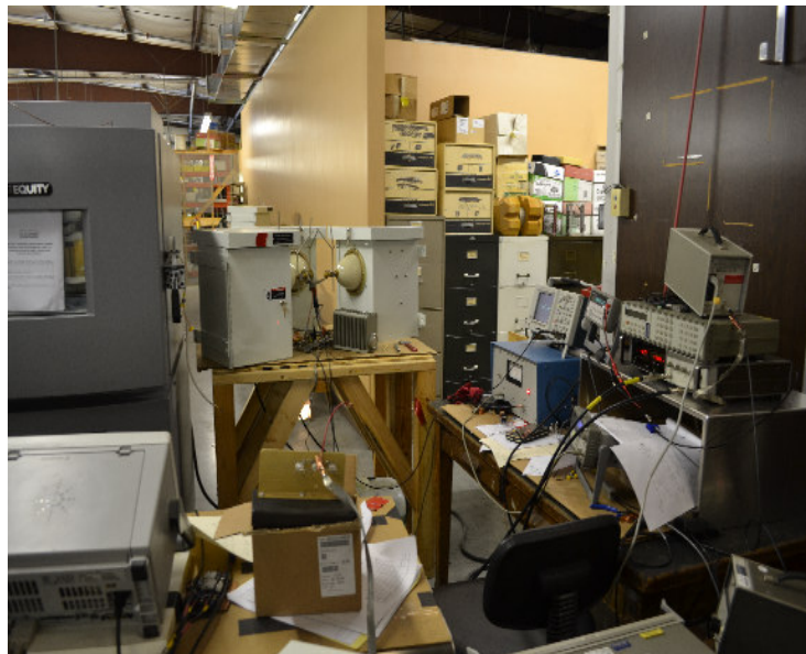
FIGURE 4. Instrumentation setup for ambient testing of the voltage sampling units.
