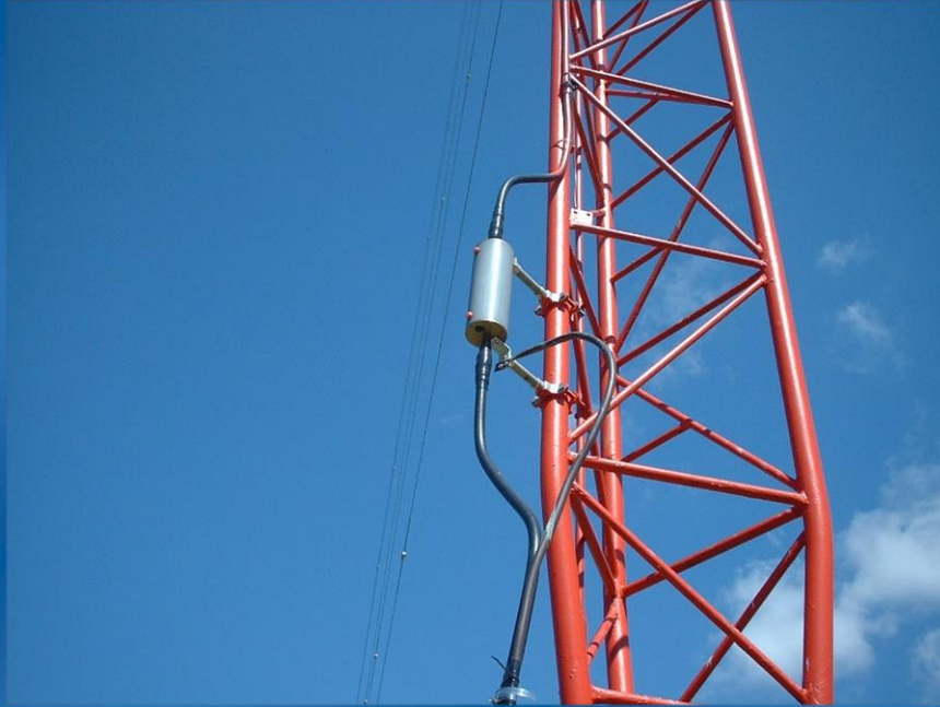
FMC-0.2P Isocoupler with included mounting brackets and standoff insulators
