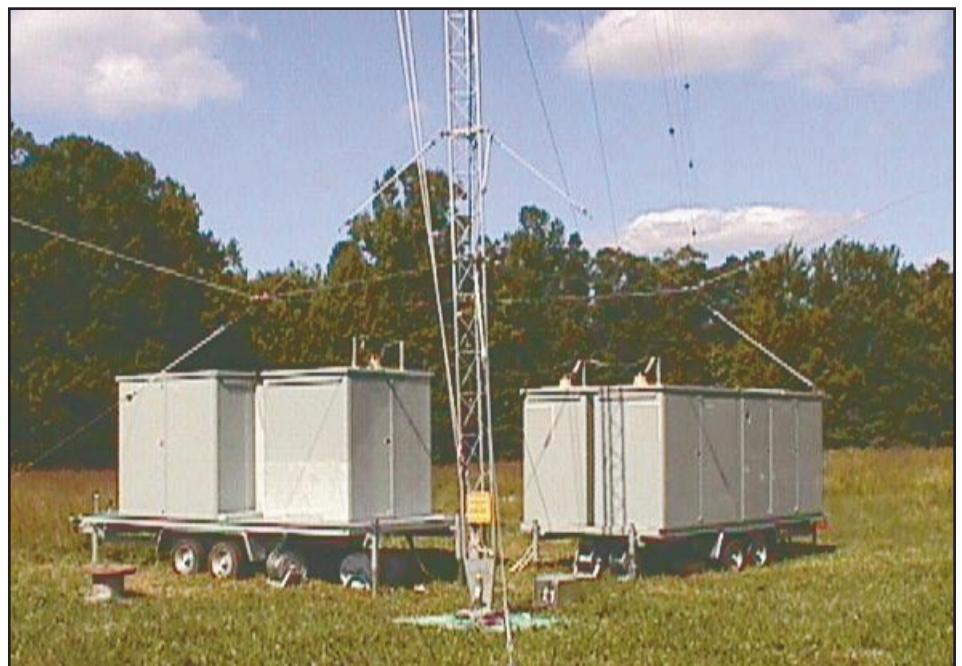
Photo 2: Mobile triplexer installed at tower base
