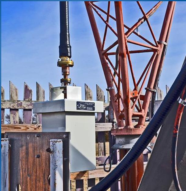
FMC-05LPTV for LPTV on AM base insulated tower
