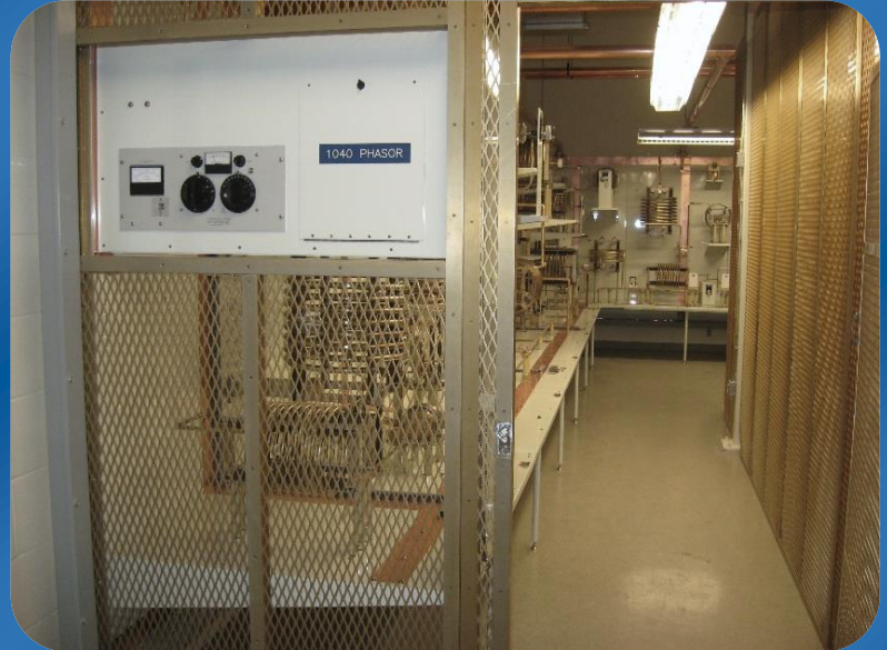
Open-panel wall-mounted phasing system with shielded partitions
