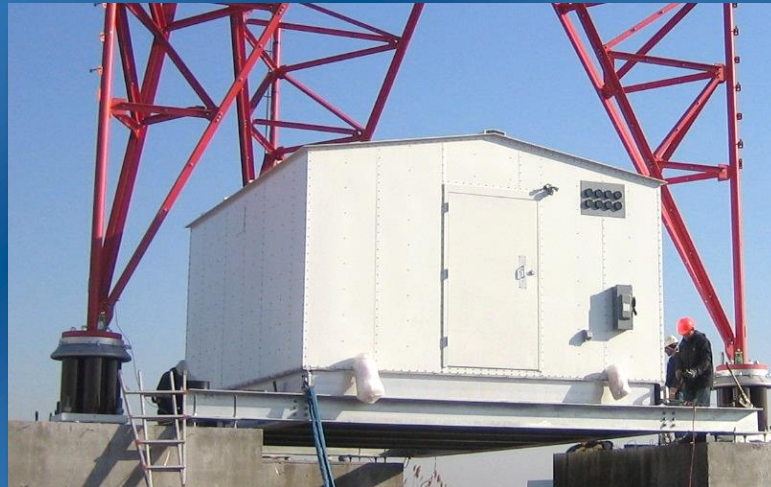
All-Aluminum pre fabricated tuning houses in which the matching and filtering networks can be installed
