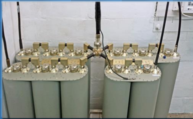
Kintronic FMC4X1.2KW supplied 4-input FM combiner
