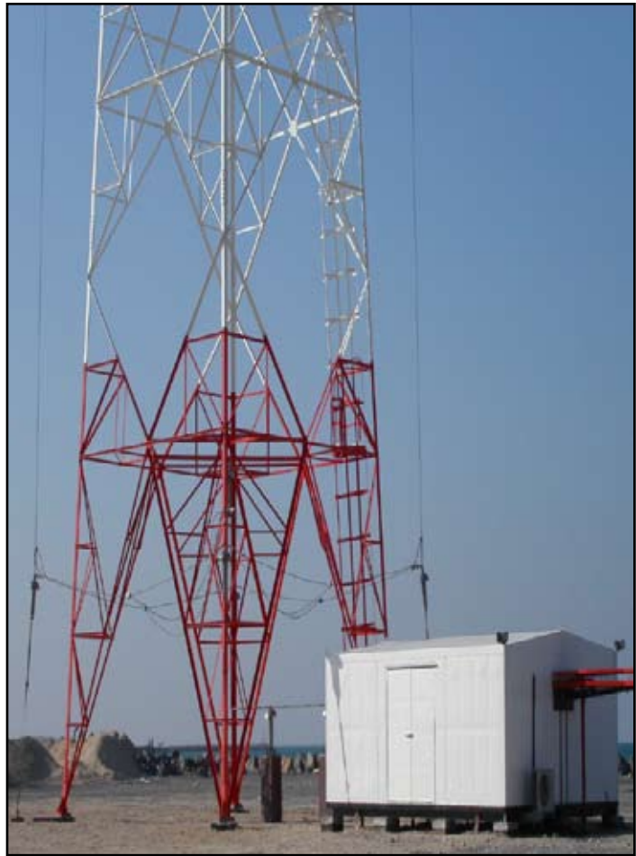
Unipole Installation on a Self Supported Tower
