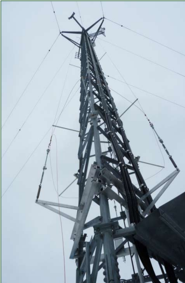
Unipole Installation on a Fixed Cross Section Guyed Tower
