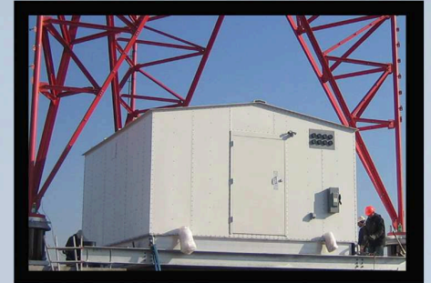
Pre-fabricated Tuning Houses or Transmitter Buildings (WEPN - New York) *installed by MIKAB CORP.
