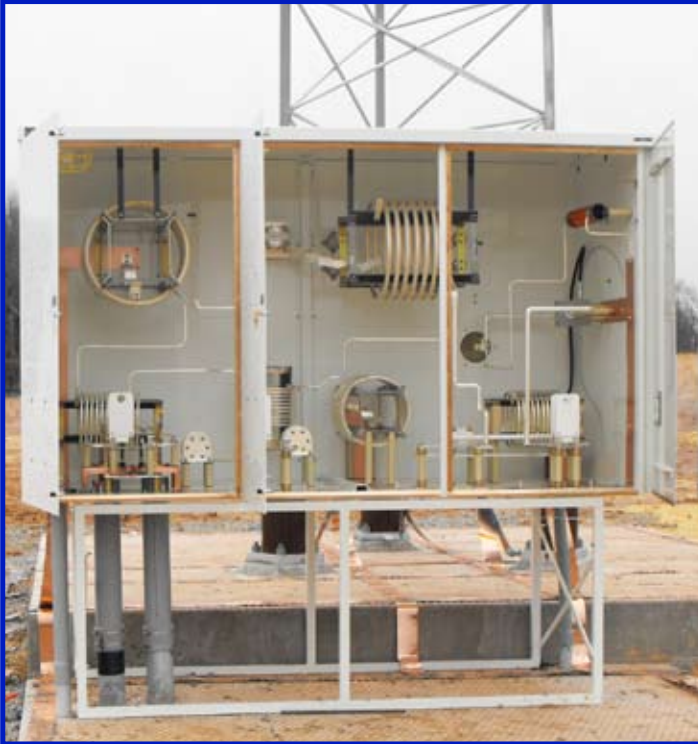
Weatherproof ATU on Optional Support Stand
