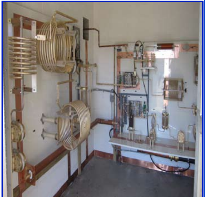
Wall Mountable Open Panel and Shelf ATU
