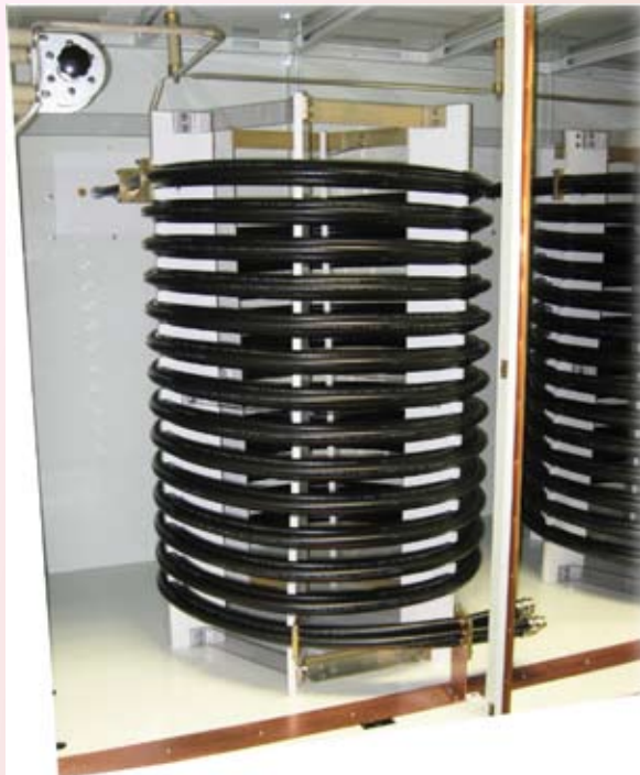
CUSTOM ISOLATION INDUCTOR CONFIGURED FOR DUAL STROBE HEAD INSTALLATION ON AM BROADCAST TOWER
