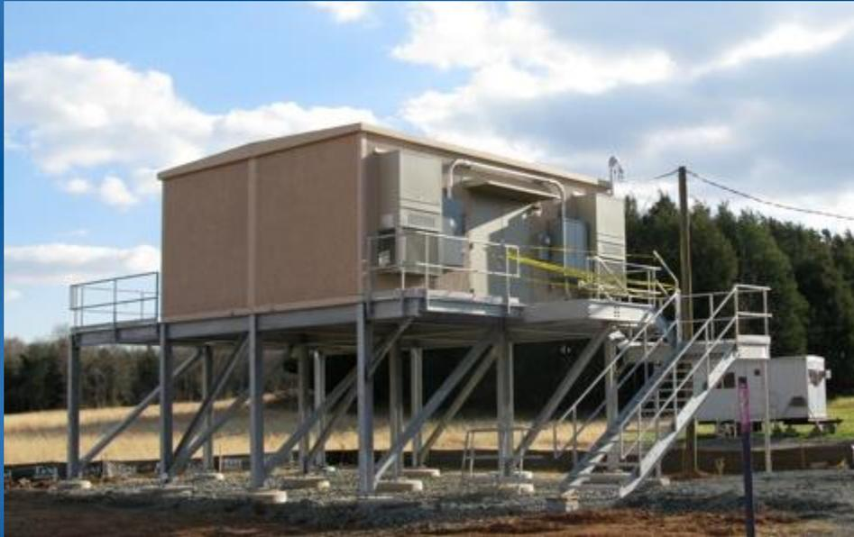
Pre-fabricated transmitter building with galvanized steel supporting structure for WAGE-AM, Leesburg, VA
