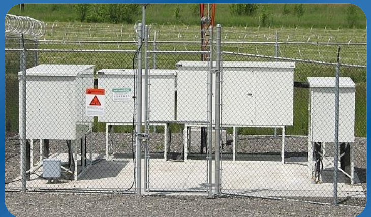
Painted aluminum weatherproof cabinets with stands configured for installation on concrete pad
