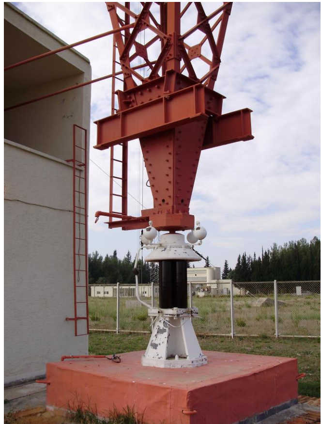
Fig 1 Typical Base Insulator, Antalya, Turkey
