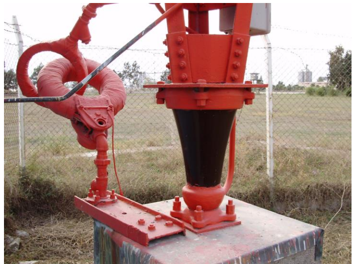
Fig 4 Typical Properly Installed Austin Transformer, Mersin, Turkey
