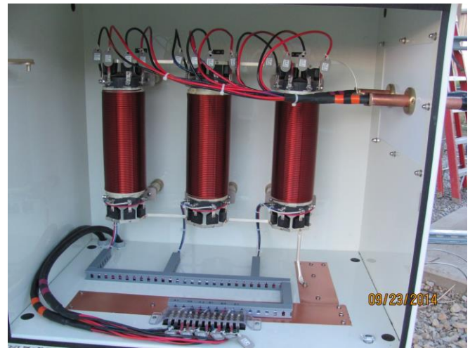
Fig 15 Multiple Lighting Chokes Provide DC Power
