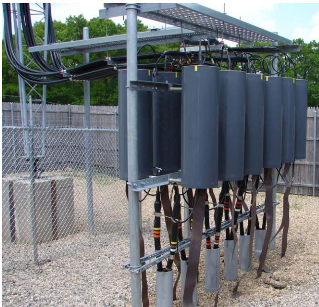
Fig 17 Typical Iso-Couplers for a Wireless Facility
