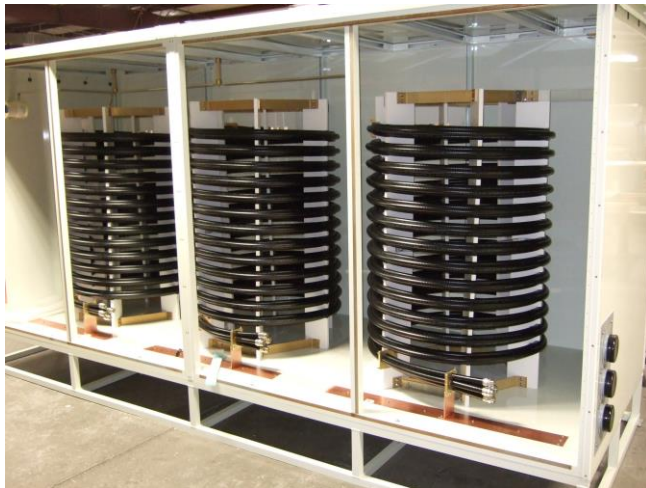
Fig 10 Iso-Coils for Wireless Facility Isolating 12 Separate 7/8 Coaxial Lines
