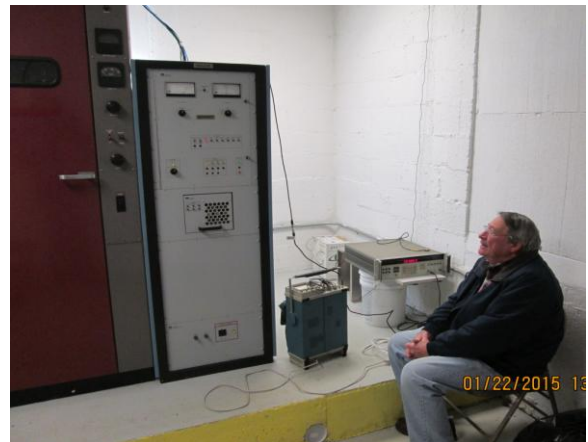
FIGURE 7. PHOTO OF THE EQUIPMENT SETUP AT WGAP
