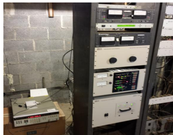
FIGURE 6. PHOTO OF THE EQUIPMENT SETUP AT WKPT
