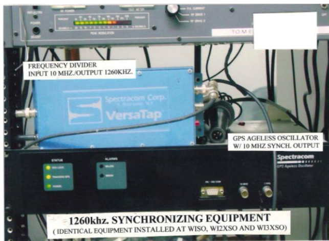
FIGURE 12 – WISO RF SYNCHRONIZATION EQUIPMENT
