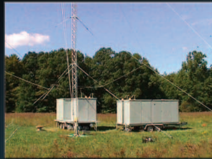
RF matching and Filter Unit on Dual-Axle Trailers
