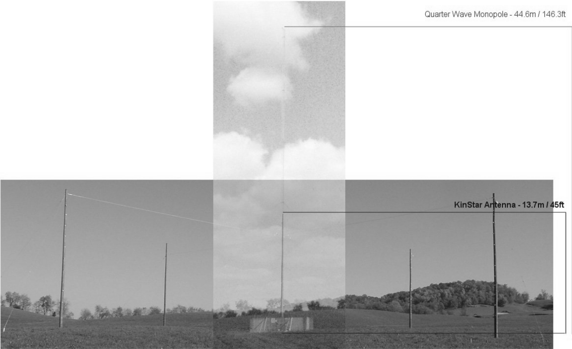
Figure 1 – Composite photograph of quarterwave tower and KinStar antenna at the WS2XTR test site, showing height comparison. Both antennas operate at 1680 kHz.
