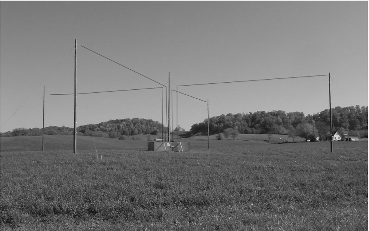
Figure 12 - KinStar antenna at WS2XTR test site. Vertical radiating and top loading wires have been enhanced for visibility. The pole structure is about 50 feet tall, and 105 feet in radius for operation at 1680 kHz to support the radiating antenna with a height of 45 feet and 100 foot radius. Each pole is approximately 55 feet long, with approximately 7 feet of that in the ground.
